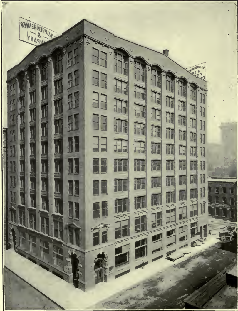
THE KENT BUILDING.
